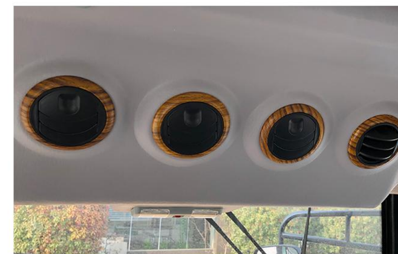
Heating and cooling air conditioning
